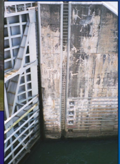
Concrete deterioration at Chickamauga
