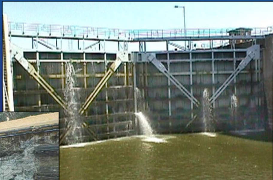
Leaking miter gates, Upper Miss Lock 19
