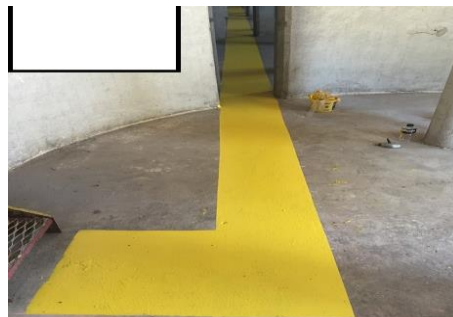
*designated walkways and working area
