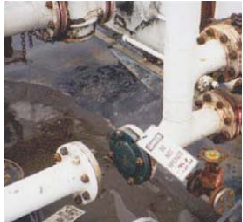
Blanking Device with Tag
